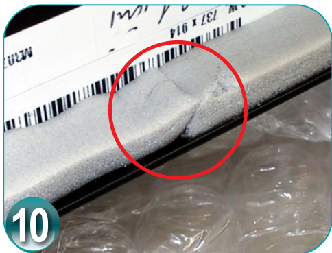
10 Apply foam tape all the way around the flange. Mid-Bottom of the window is a suitable starting point. Take particular care around the four radius corner. Cut off tape end at the starting point to form a continuous seal. Join foam tape, cleanly, as above.
