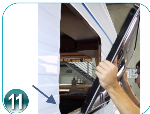
11 Fill Seams with silicone - then crush. Position window in opening on the wall of the van where it is going to be permanently installed. Do this from the outside of the van. Note! Bottom of the window to go in first - to clear locks.
