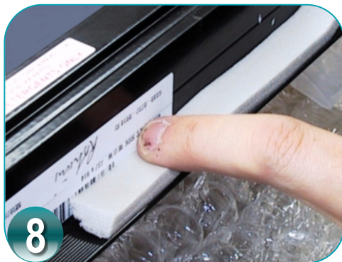
8 Clean dust and dirt from around the opening where the window is going to be fitted. Wipe window main frame flange with a dry cloth to remove dust. Apply bedding compound to flange. Foam tape is used in the case of the above picture.
