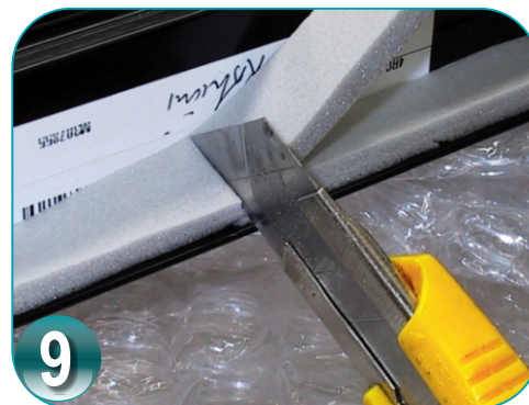
9 For bedding compound use: 1). Butyl Rubber Tape. 2). Double sided or one sided foam tape. 3). 100% silicone rubber sealant. 4). A suitable combination of the above. DO NOT USE AN ADHESIVE
